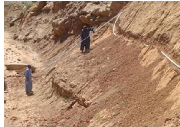
Laying down water pipelines, Balochistan
